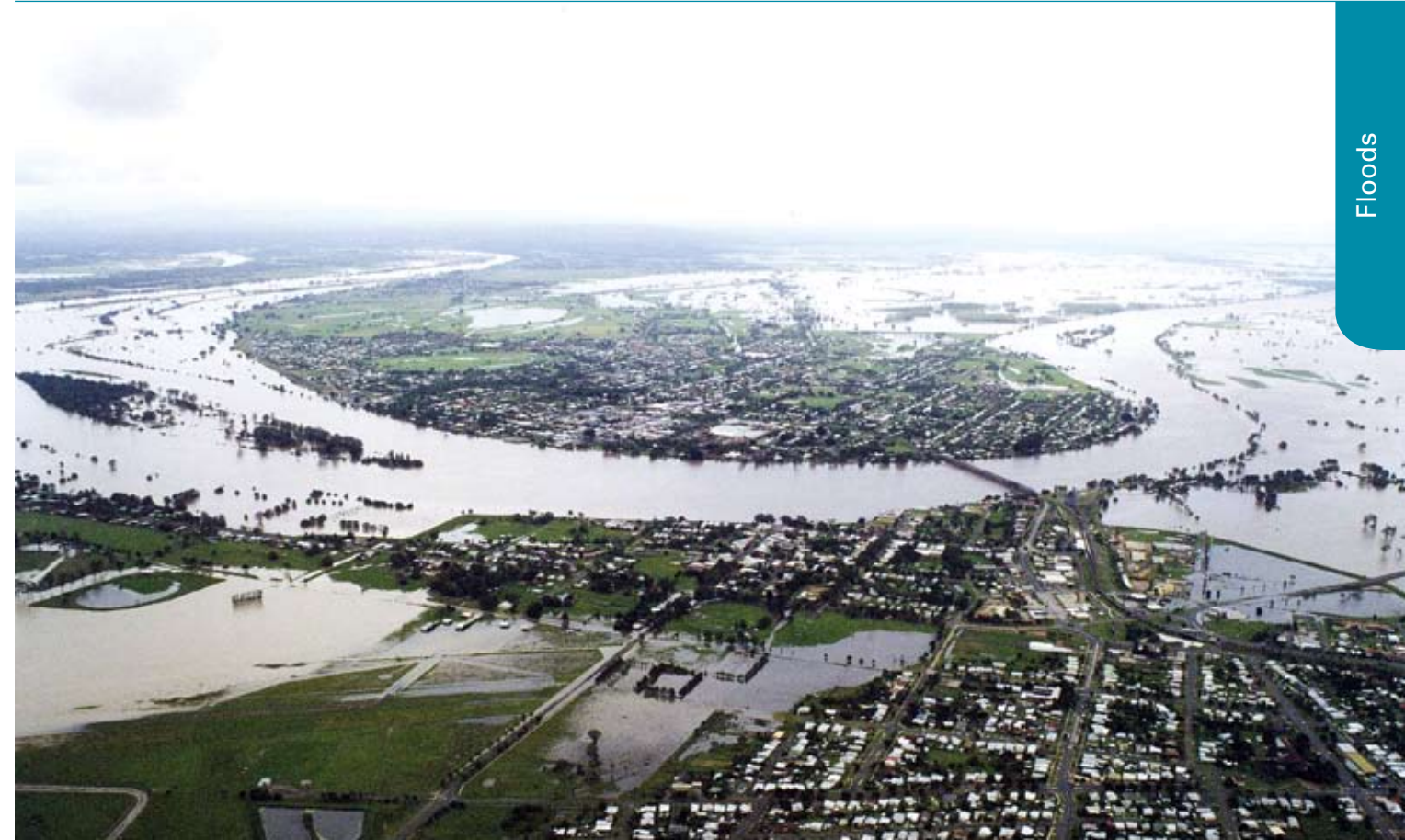
IMAGE: Grafton and South Grafton, March 2001 floods (courtesy of Clarence Valley Council)
