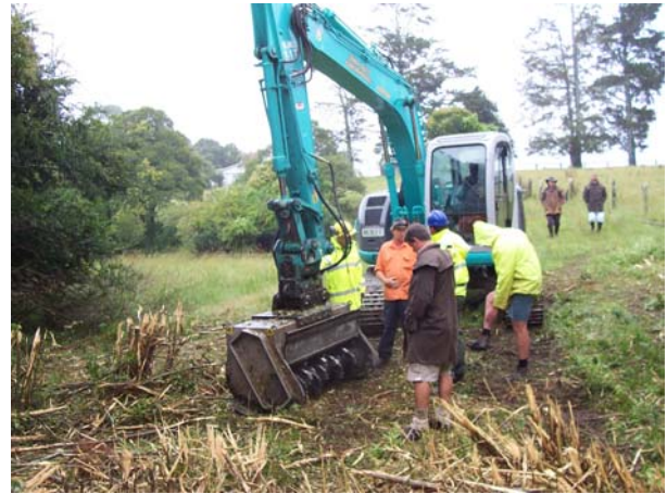
Excavator-mounted mulcher trial at North Dorrigo, mulched privet stumps in foreground
